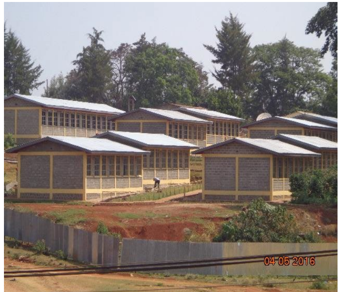
Figure 2. One of the schools constructed by SSD
